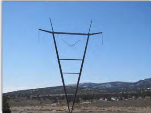
SWIP Project 500kV AC Guyed-V
